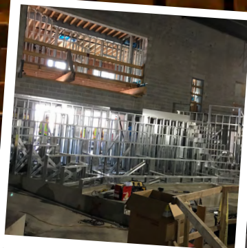
The bones of the Mike & Bobbie Voris Mainstage theatre under construction!
